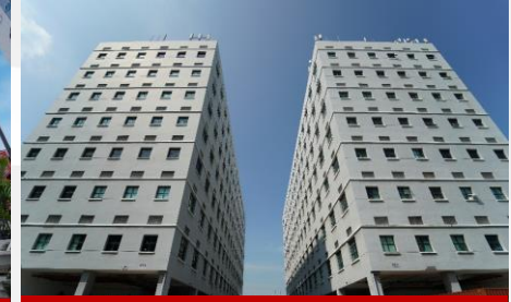
Citilink Warehouse Complex
