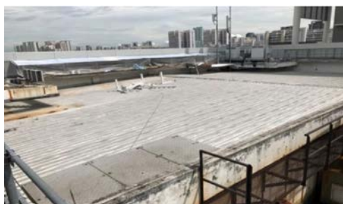
Metal roof top available for solar installation
