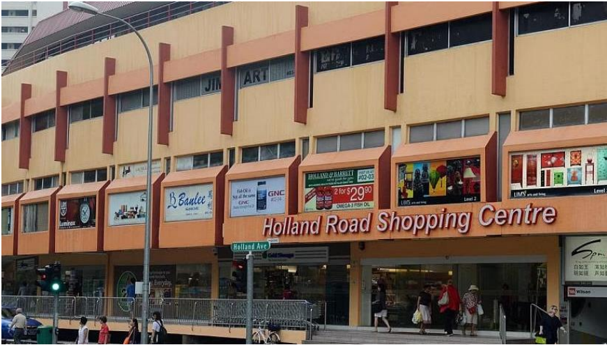
Holland Road Shopping Centre retail space and car park
