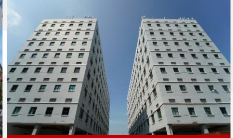
Citilink Warehouse Complex
